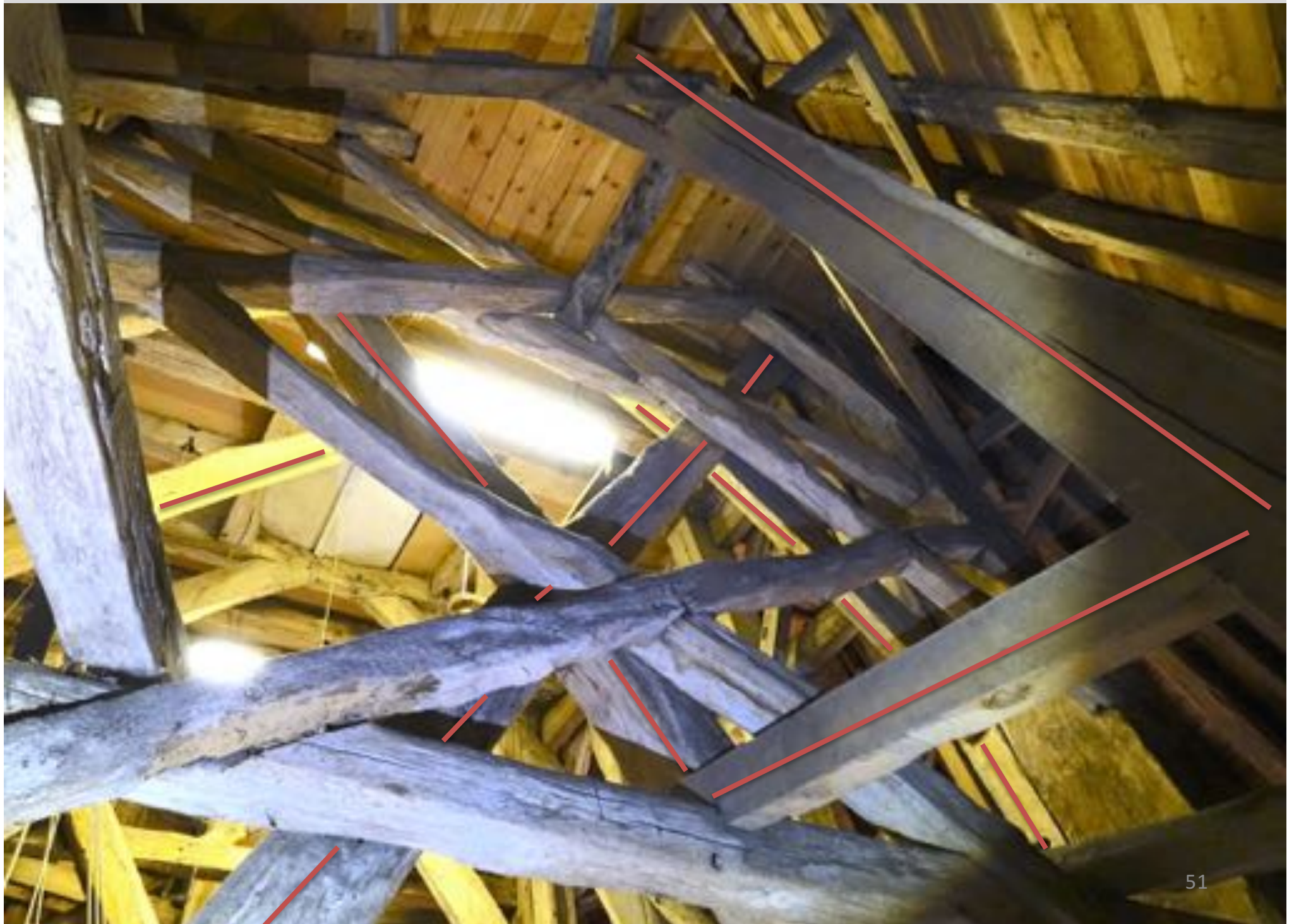
The older tower seen from its former outside. Red lines mark the new added tower construction.
