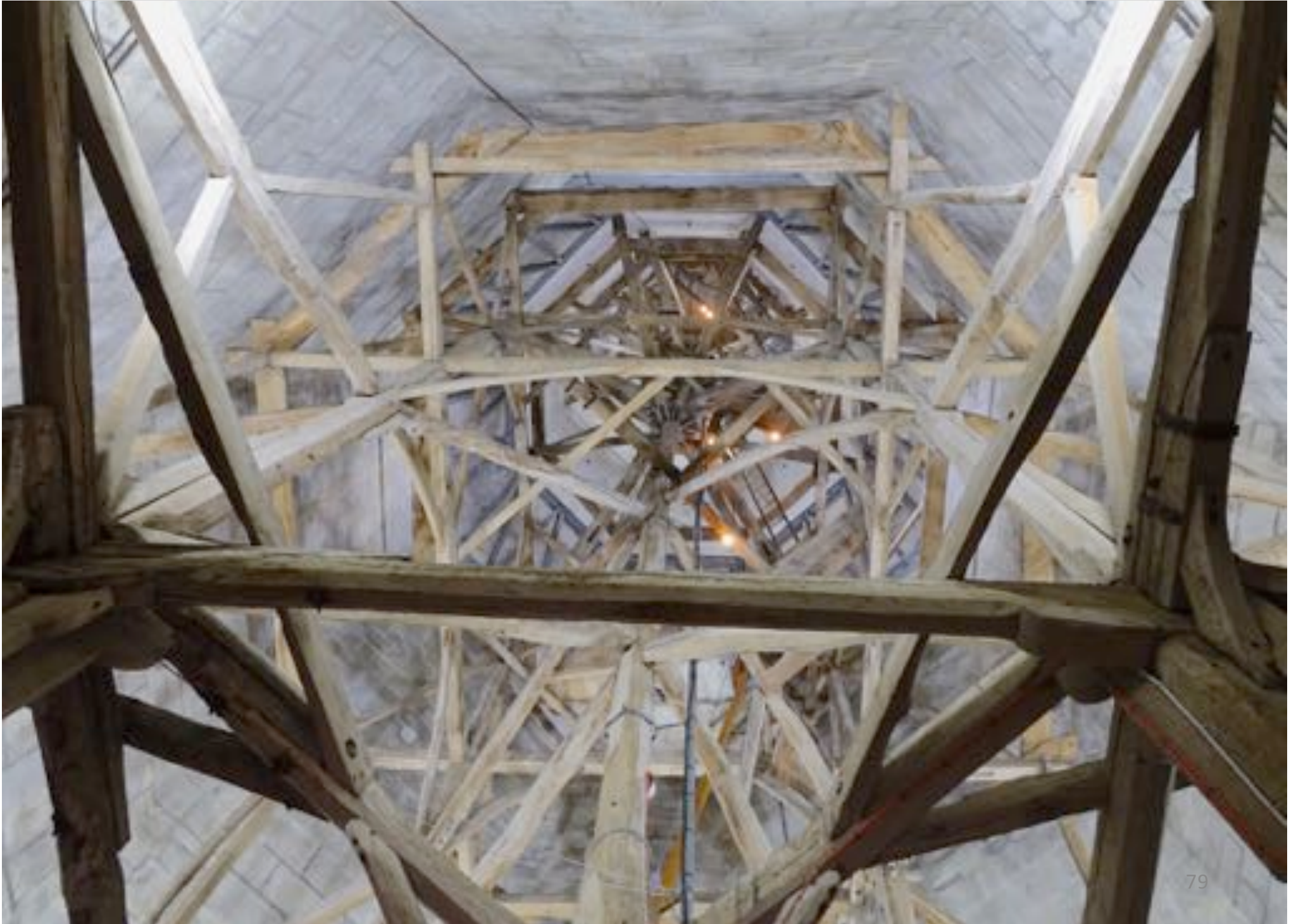
Scaffolding inside the stone spire. Some wood is changed in modern time.
